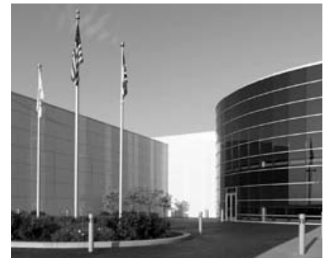
Dana Corporate Offices and Technology Center – Maumee, OH, USA
