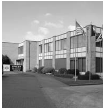
Dana Brugge Facility, Belgium
